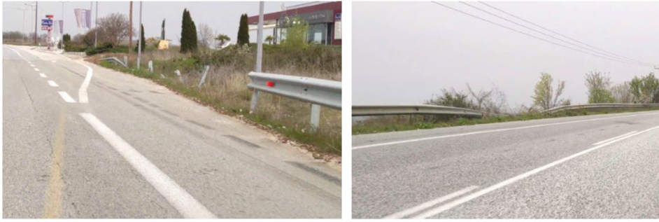
Figure 7: Damaged restrained systems.
