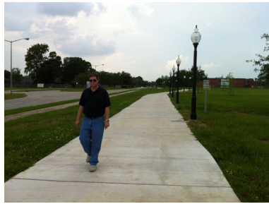
Figure 3: Post-installation view of pedestrian and bike path with acorn-style pole fixtures and pavement surface LRV of 39%.
