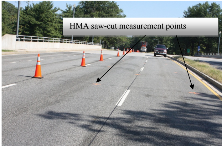
Figure 3: Saw-cuts treated pavement joints.
