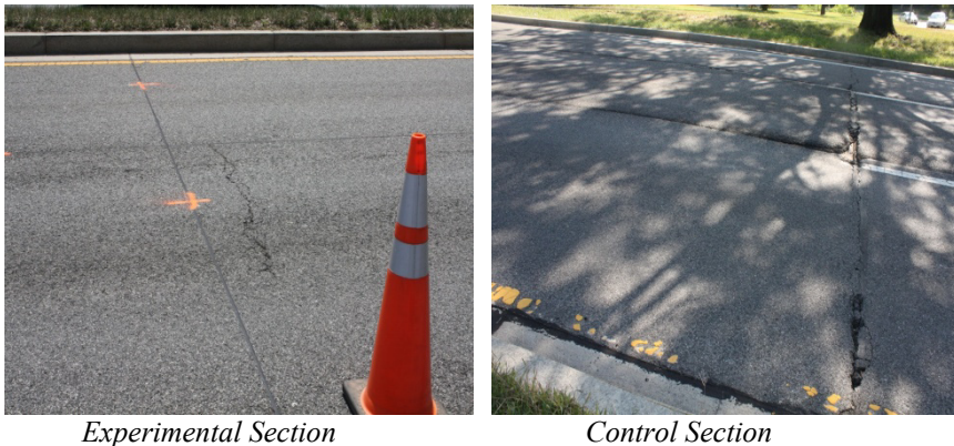
Figure 4: Visual inspection of experimental and control sections.
