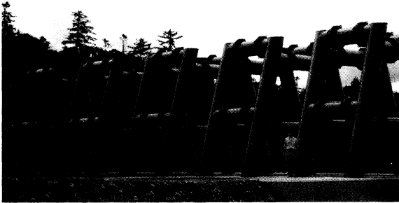
Photo 1 : B-type slit dam
