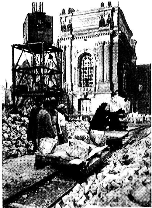
Fig. 5. Frauenkirche in Dresden, loading of the „rubble carts“ during the initial archaeological clearing of the ruin, 1948
