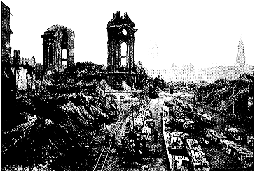
Fig. 6. Clearing work on the Muenzgasse with a view of the ruins of the Frauenkirche, City Hall, and the Church of the Holy Cross, the latter of which are being restored, 1952
