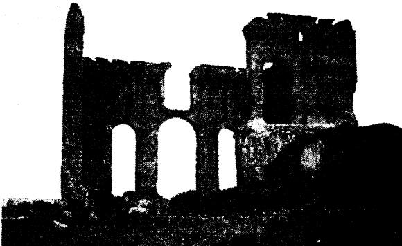
Figure 4 Façade characterised by collapse happened between 1910 and the eighties
