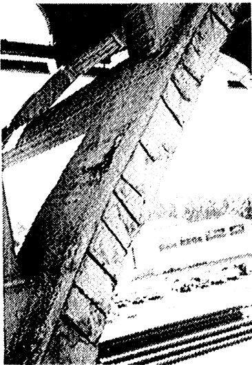
Figure 4: Exposed reinforcing
