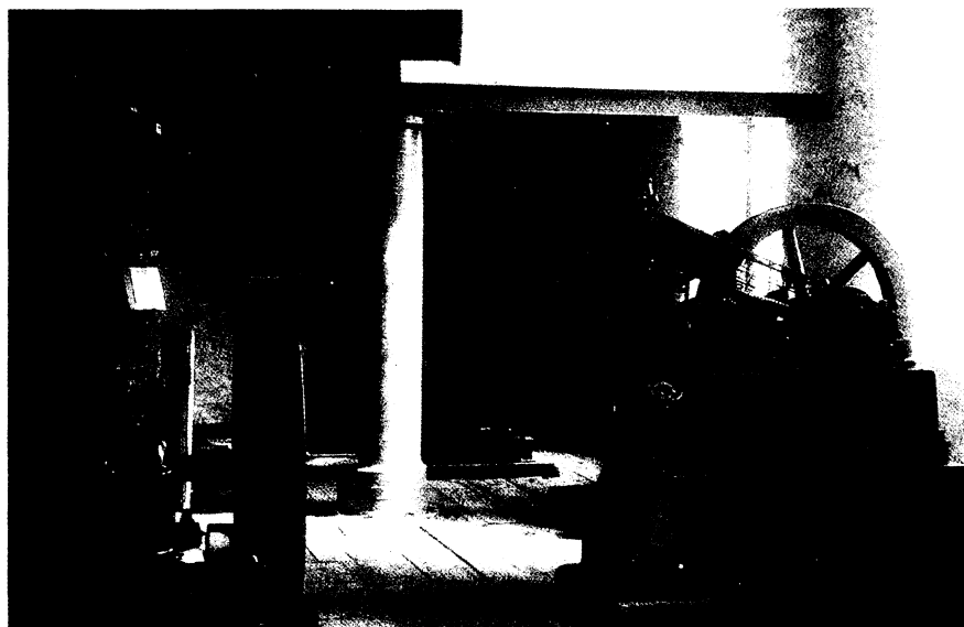
Figure 4: Interior of Engineering Workshop Showing Gas Engine in the Background and the Steam Engine on Right.
