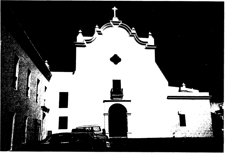
West Facade - San Jose Church
