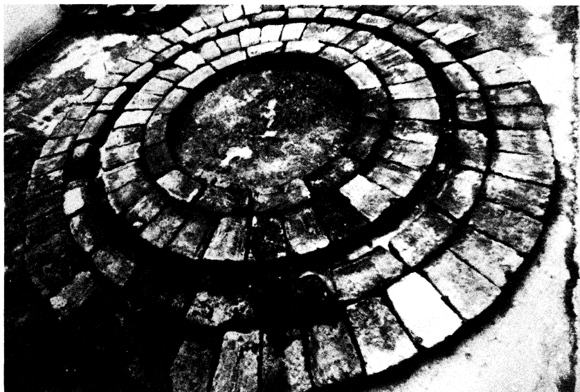
Figure 4: Reconstruction of the cross section through a typical double-stack chimney (Settimo Torinese, originally a tanning plant).
