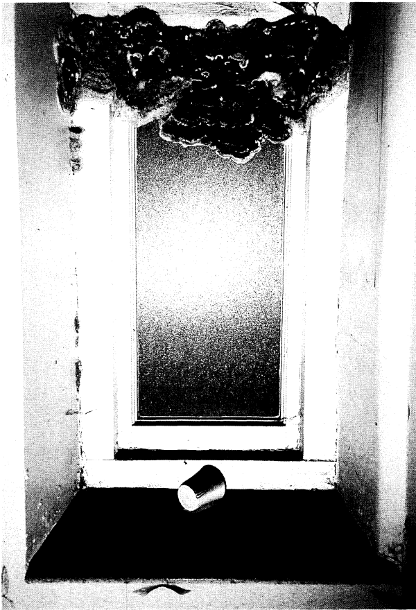
Figure 2 Dry rot fruiting body
