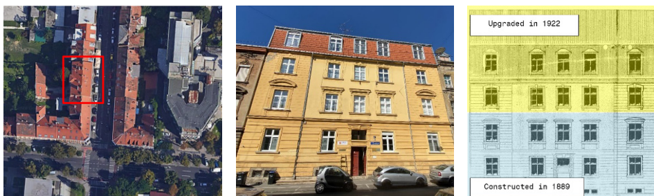
Figure 5: Case building for the simulation of retrofitting and reinforcement levels, Kačićeva 22, Zagreb, Croatia [17].
