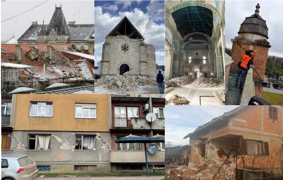
Figure 2: Damage to masonry structures. (Source: Authors.)
