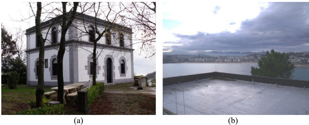
Figure 4: (a) General aspect of the building today; and (b) Current flat roof.
