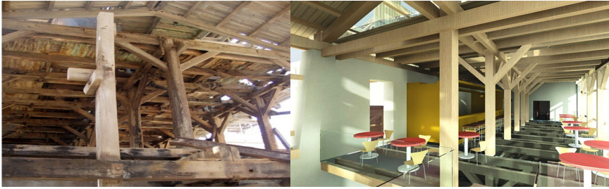
Figure 5: Current state and design for the interior spaces of the Washery.
