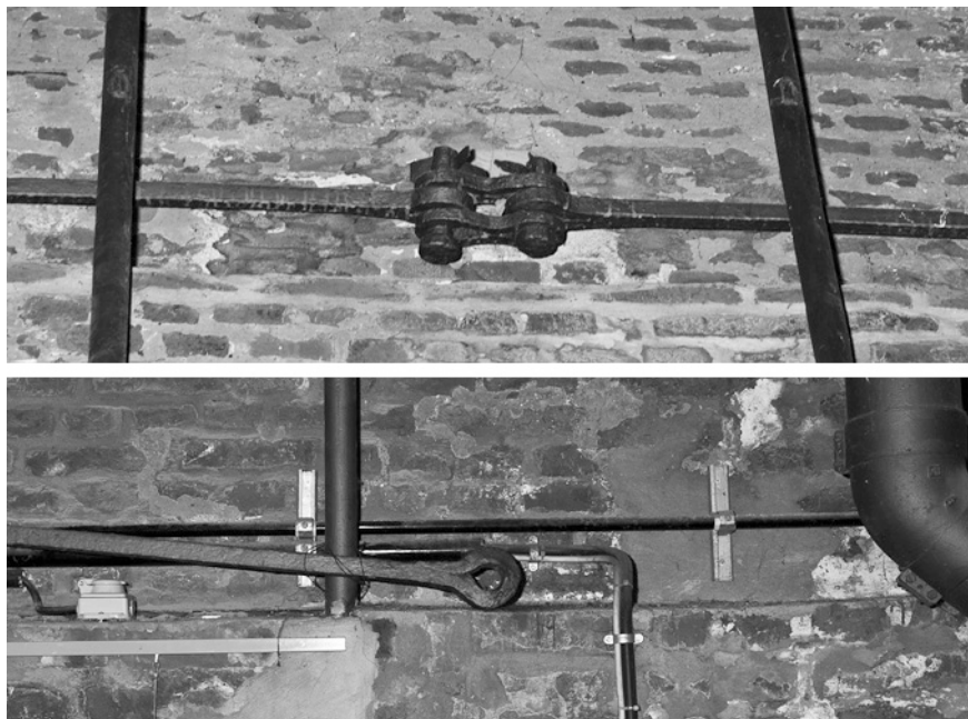
Figure 3: Tie at the original state and on the opposite side.
