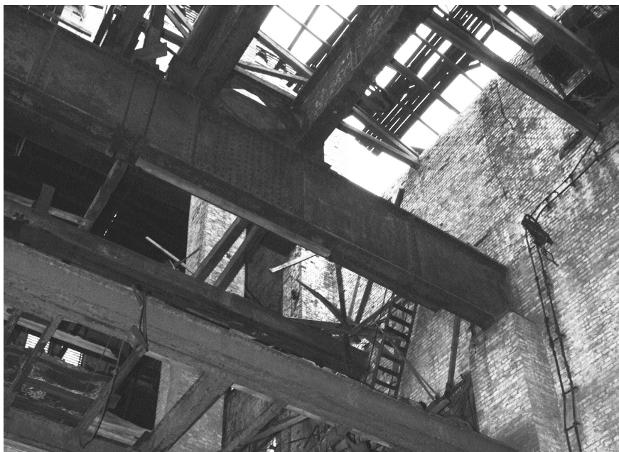
Figure 5: Partial demolition at Ernst Schacht IV.
