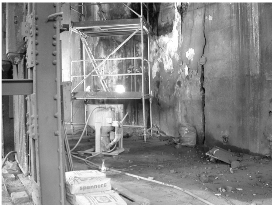
Figure 6: Needling and concrete injection at masonry cracks.
