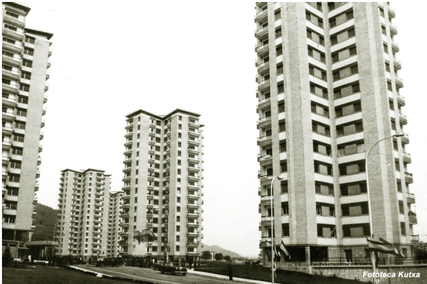
Figure 3: Photograph of the Bidebieta Towers.
