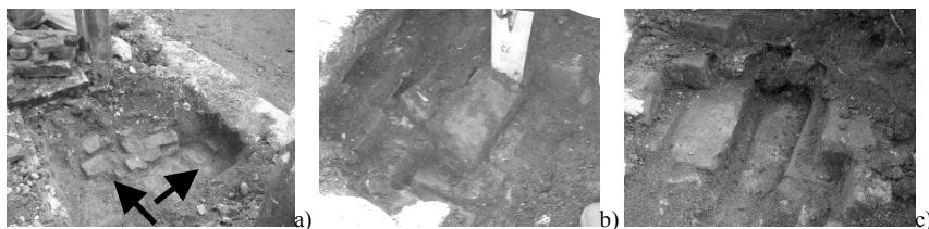
Figure 6: a,b,c: Ditch T1: the sequence shows two masonry leaves, one behind the other.
