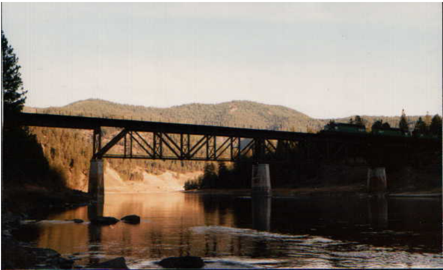
Figure 6: Montana Rail Link Bridge, Paradise, Montana over the Clark Fork River.
