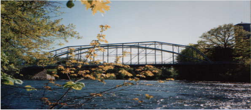
Figure 5: Rehabilitated Stuyvesant Falls Bridge for HS-20 Loading.
