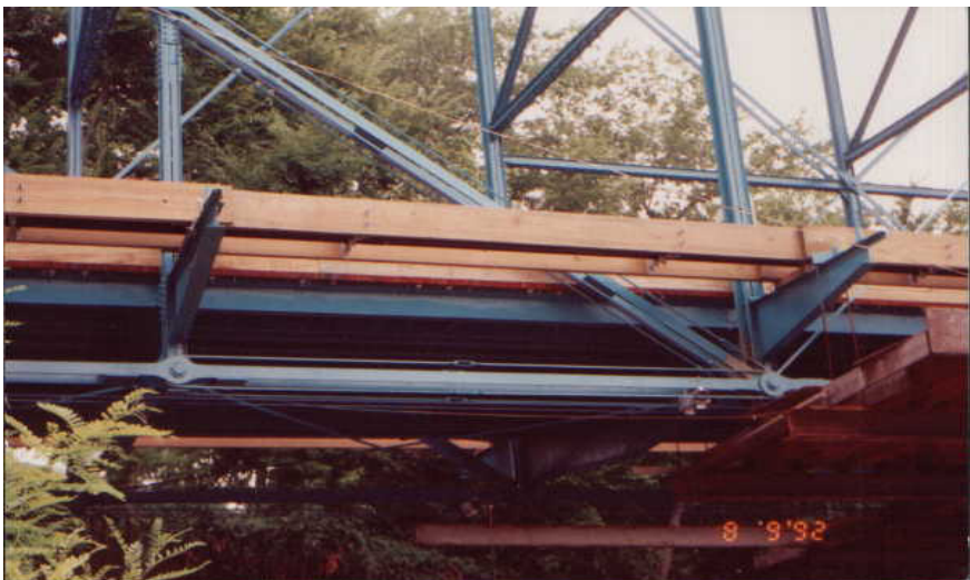
Figure 2: Several posttension bars looped around one common pin – conventional rehabilitation.
