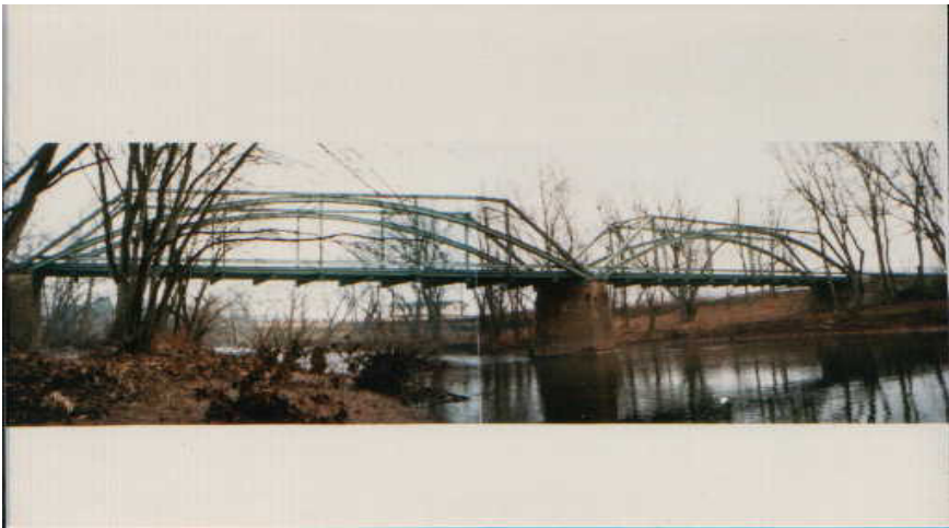
Figure 9: Worthington Bridge, Douglas County, Oregon (over the Little Umqua River).
