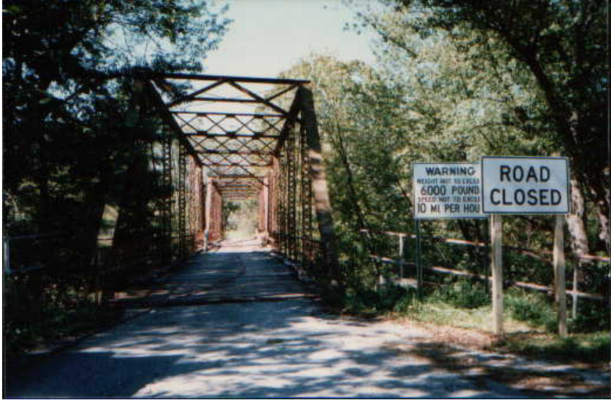
Figure 8: Mumma Ford Road Bridge, Carroll County Maryland (over the Monacasy River).
