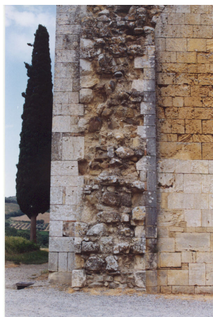
Figure 1: An example of multi-leaf masonry wall (St. Antimo Abbey, Tuscany, Italy)
