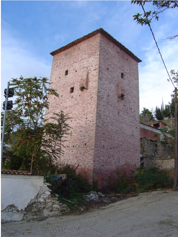
Figure 4: The Tower of Mamjios in Tsaritsani, with its battlements and loop-holes, on the outskirts of Larissa.
