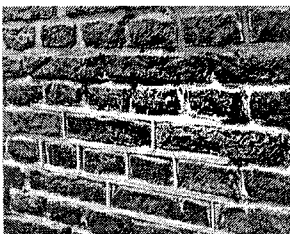
Fig.5 Spaarndam (NL), 'Rijnlandhuis', historically wrong pointing (test panel)
