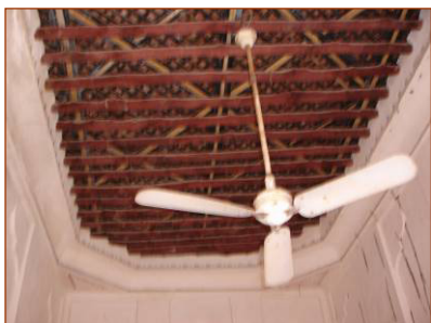
Figure 4: Exposed roof structure.
