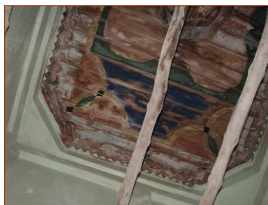
Figure 5: Colored wooden roof.
