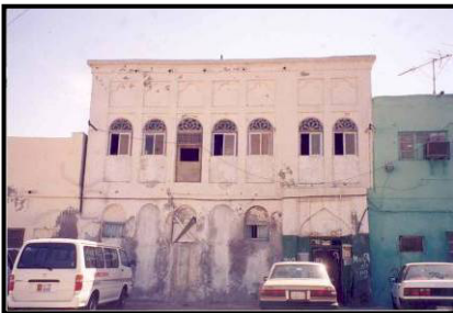
Figure 8: Front elevation (before renovation).
