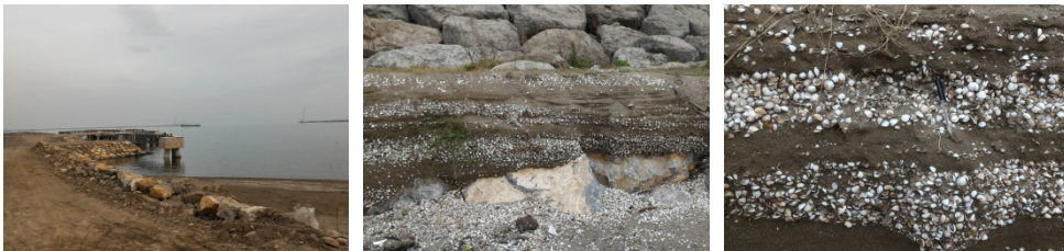
Figure 5: Typical coasts of the Constructed Trade-Industrial Free Zone.
