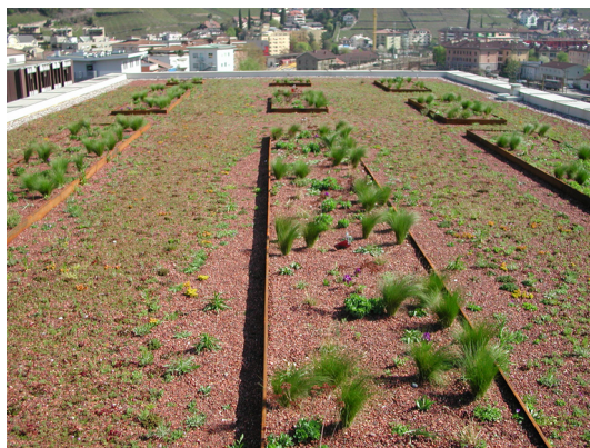
Figure 2: Integrated application of technologies for management and collection of rainwater. Calculation of the coefficient of runoff of water and the achievement of minimum standards of permeability that could be required for each industrial building.
