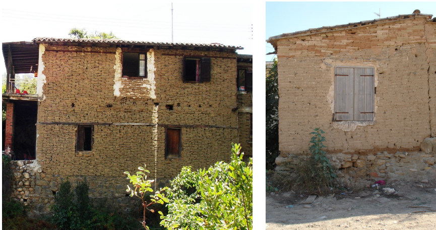
Figure 1: Local traditional buildings with load bearing walls composed of adobe masonry.
