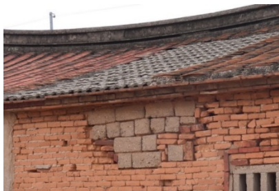
Figure 3: The mixed use of cement tiles and hollow bricks for conservation in the 1950s.
