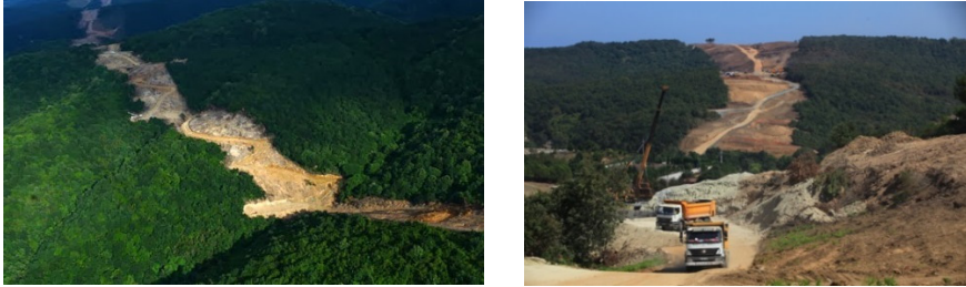
Figure 6: The Third Bridge building site view.
