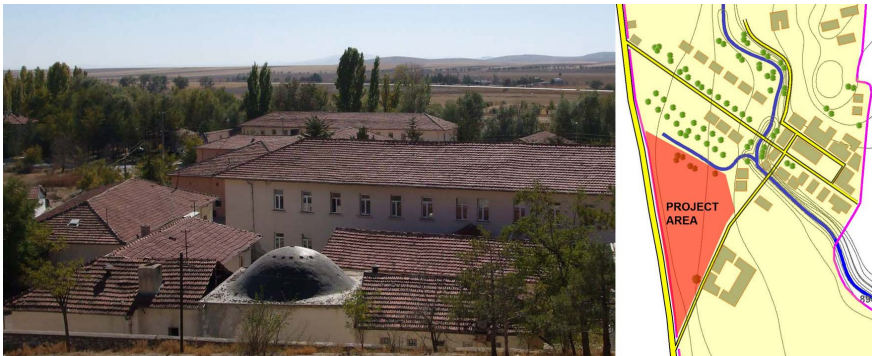
Figure 1: The Village Institute buildings with the project site.
