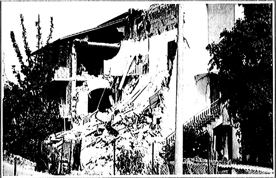
Figure 4: Partial collapse of two-story building in the settlement of Annifo.
