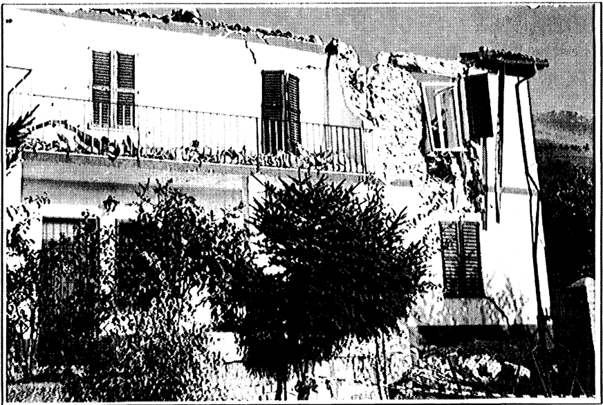
Figure 3: Collapse of the two-story building rubble masonry, in the settlement of Cesi
