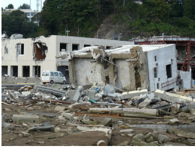
(a) Damaged building in Onagawa City
