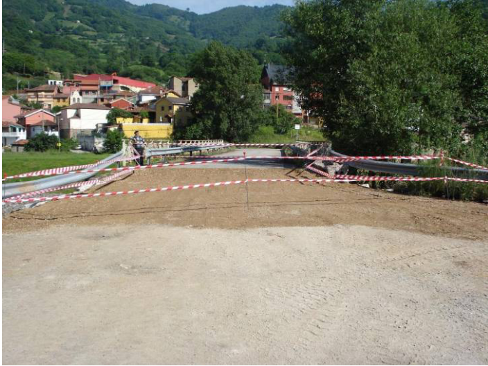
Figure 3: The same road, after TRAGSA intervention.
