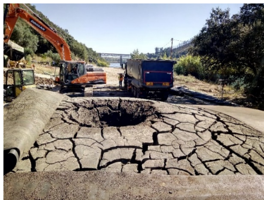
Figure 6: Removal of the dewatered bag content.
