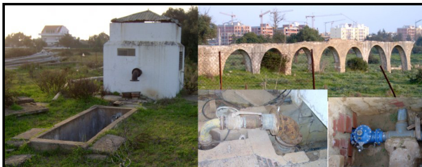
Figure 3: Abandoned sluices, pumping stations and boreholes (São João da Ourém, March 2006 – Photos by José P. Monteiro).
