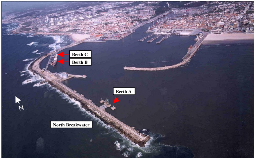
Figure 1: Location of berths A, B and C of Port of Leixões oil terminal, APDL.
