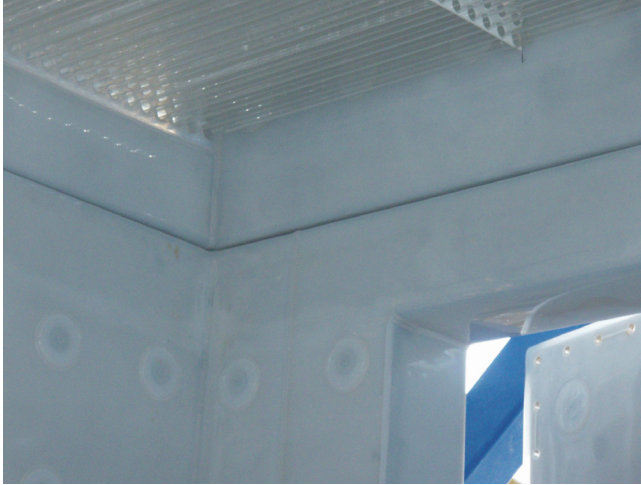
Figure 4: Gas/gas condensing heat exchanger. The gaseous heat transfer media runs through glass pipes. Courtesy Panergetic AG, FL-Schaan.
