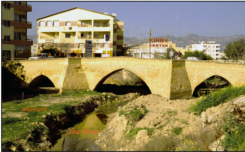
Figure 7: The Mintzeli or “Venetian Bridge” was constructed for commerce to Kyrenia across the arroyo of the Jinar/Almyros River north of Orta Keyu. Modern sediment against the bridge piers suggests that the flood plain deposits are at least 2m thick.
