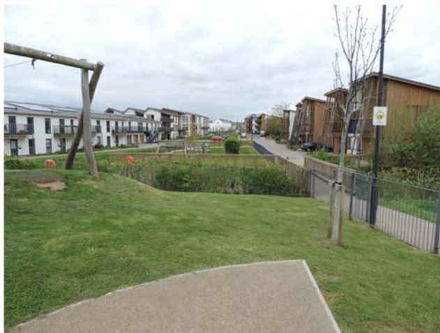
Figure 6: Hanham Hall swale site visit, May 2017.
