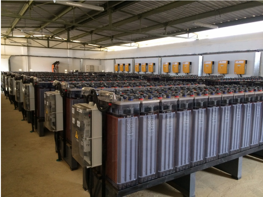
Figure 8: Photo of the battery room, the clusters and multicluster system.
