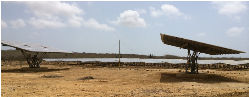
Figure 9: Photo of the isolated photovoltaic installation. View of the solar trackers and fixed installation.
