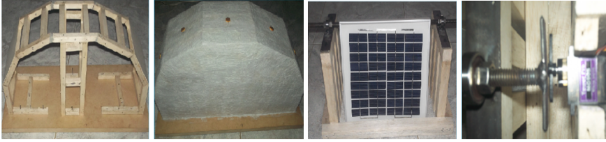
Figure 5: Details of the construction process.
