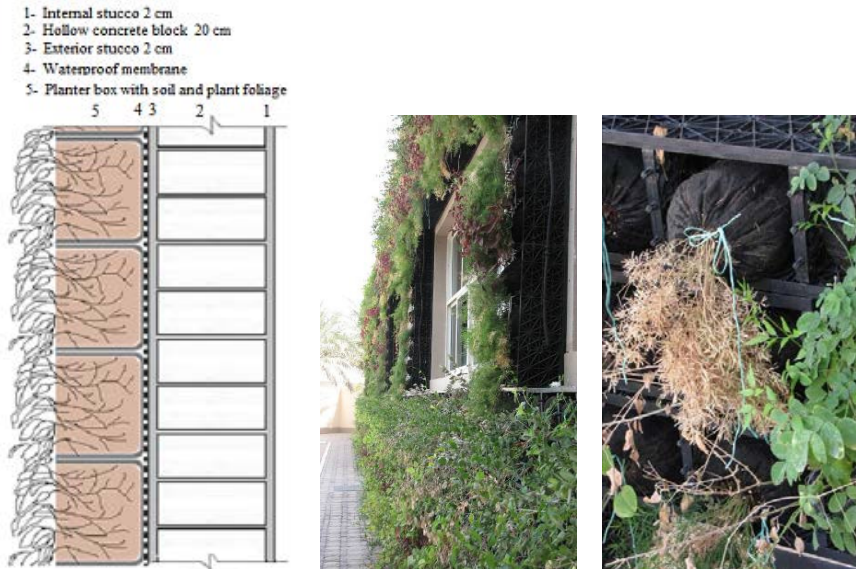
Figure 3: Installed living wall system, Liwa International School, Al-Ain.
