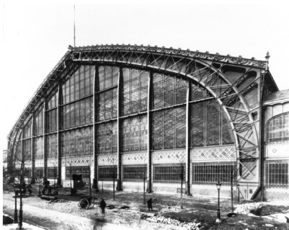
Figure 7: F. Dutert: Galerie des Machines first three point arch (statically determined structure) [2].
