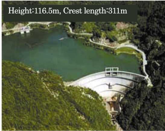
Figure 5: The Shintoyone Arch Dam.
