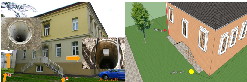
Figure 1: Location of infiltration shafts near building PK6
