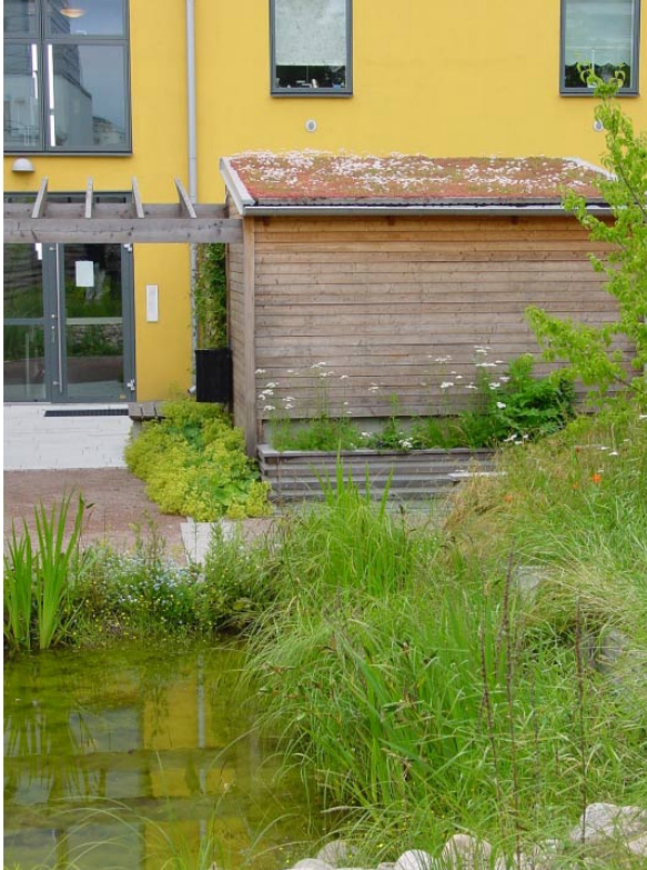
Figure 4: A pond with regional wetland vegetation in a yard at Bo01. In the background a green roof.
