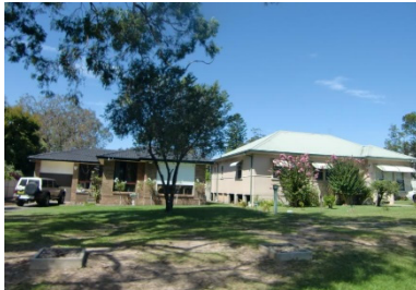
Figure 4: Private housing in Rathmines Park.
