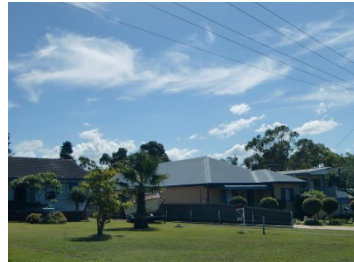
Figure 5: Private housing in Rathmines Park.
