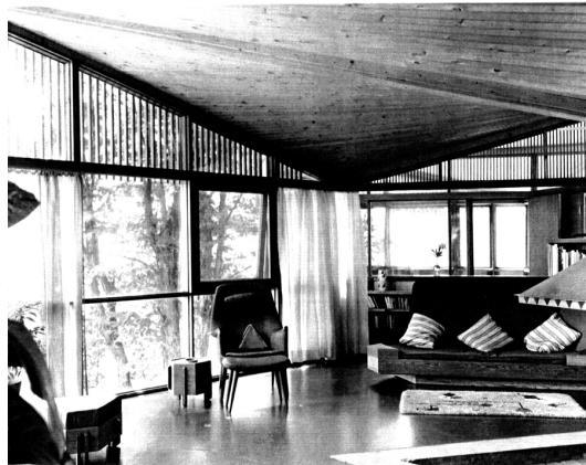
Figure 2: Strutt House – self supporting rhombi & hyperbolic paraboloid roof 1956 [7].
