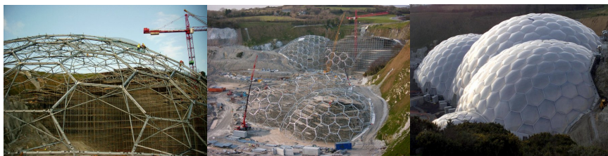
Figure 9: Eden Project, Cornwall, GB , Nicholas Grimshaw Architects, Anthony Hunt Associates engineers, structure: MERO Membrane ETFE-Pillows diameter 9 m, Dimensions: 15 590 m 2 , 100 m x220 m height 55 ( www.anthonyhuntassociates.co.uk ).
