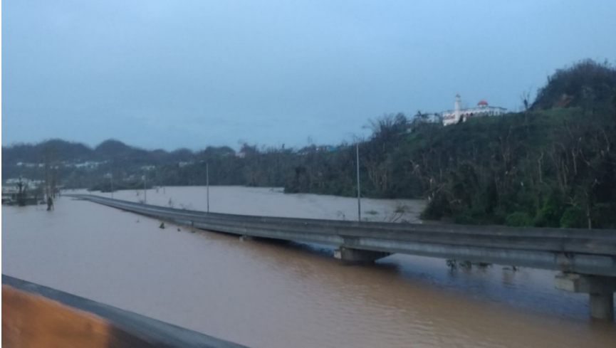
Figure 3: The flooded interchange between state road PR#2 and expressway PR#22 in the town of Vega Alta.
