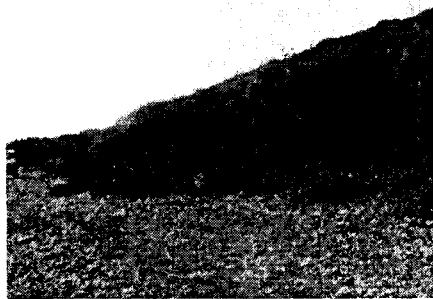
Photo. 2. Slope failure (soil falls) in silty-clay soil (old slide material) at kyria location, Proskynites coast, Rhodope.
