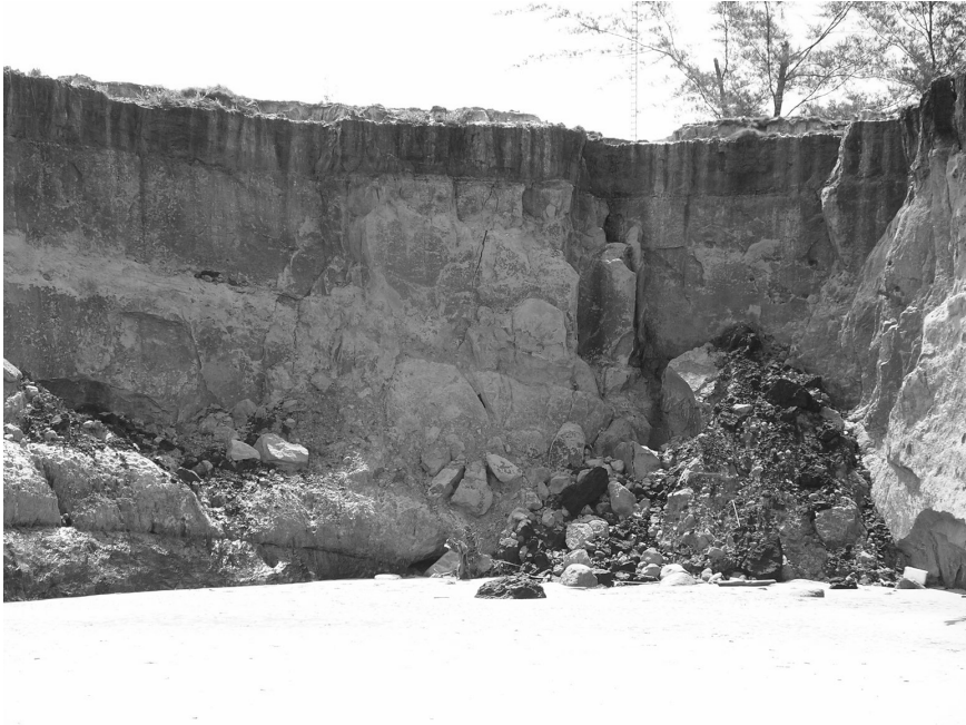
Figure 2: Typical cliff erosion along the Brunei coast.
